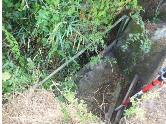
Dilapidated Upstream Sluice
