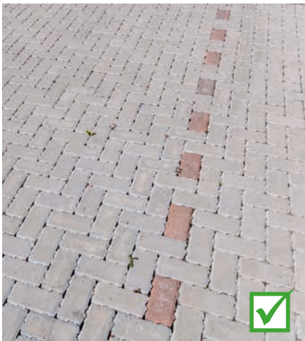
Different coloured paving should be used to demarcate the function of the space
