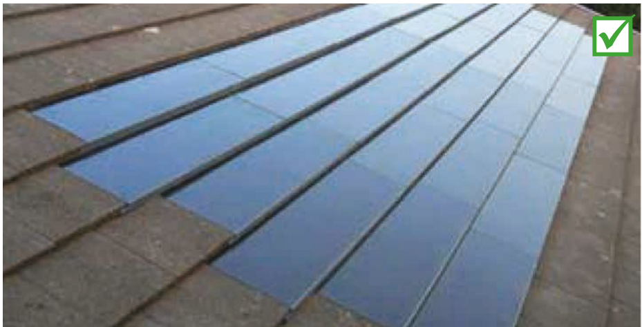
These solar slates are integrated into a tiled roof and are virtually hidden when viewed from the street
