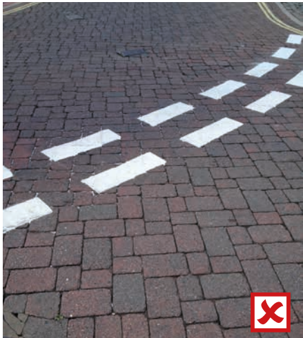
There should be no block paving where white lining is required
