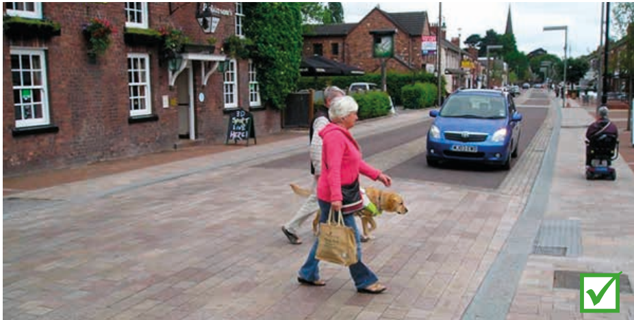
Raised shared surface crossing act as speed restraints and also assist frame and wheelchair users and people pushing buggies
