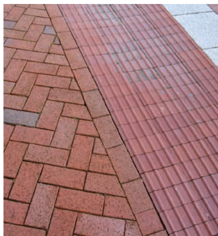
Tactile paving for partially sighted/blind users
