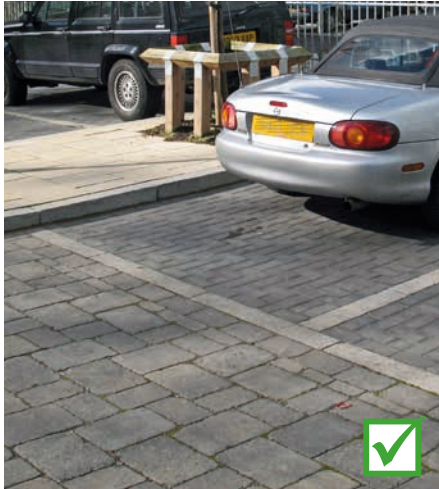
Different coloured paving should be used to demarcate the function of the space
